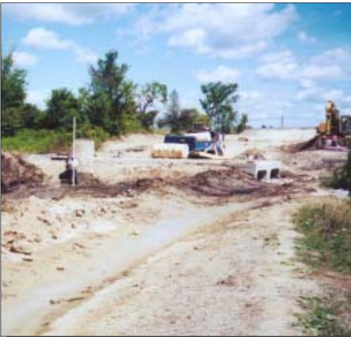
Precast concrete culvert with transition slab
