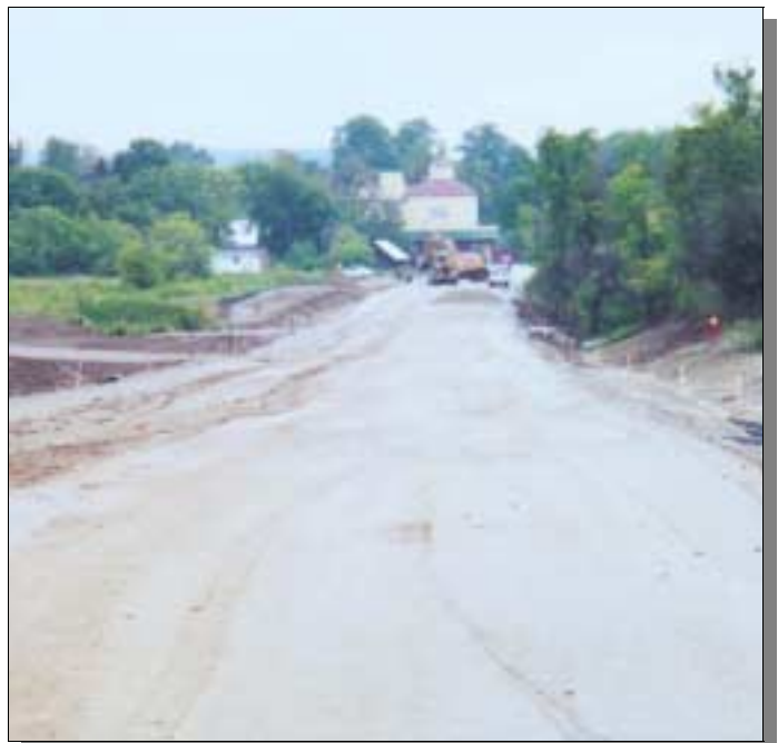
Completion of Doctor Kay Drive road base
