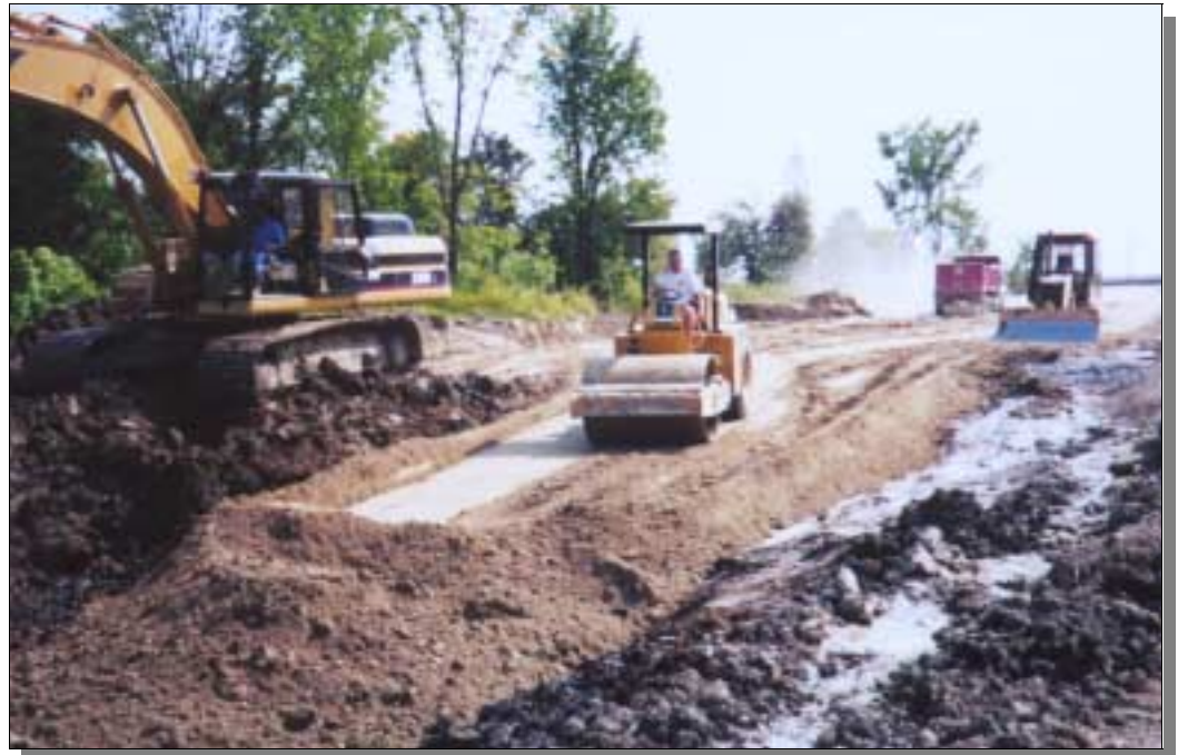
Challenging site conditions for construction of Doctor Kay Drive
